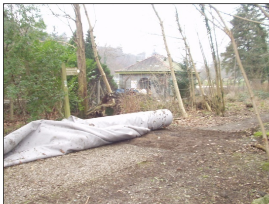
Photo 2- laying of Fibretex material onto existing subgrade
