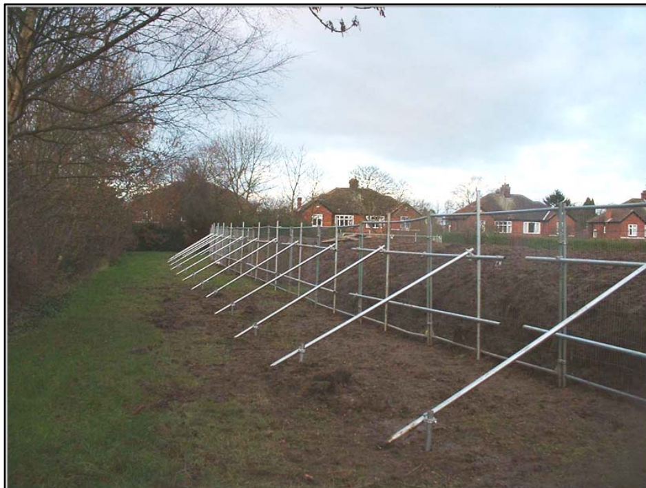
Figure 2- Actual barrier erected on site
