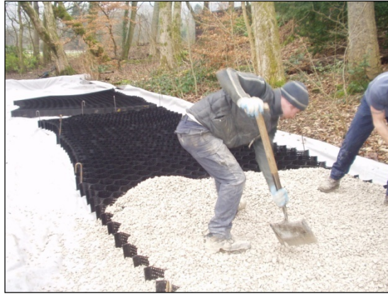
Photo 3- expanding and filling the Cellweb system
